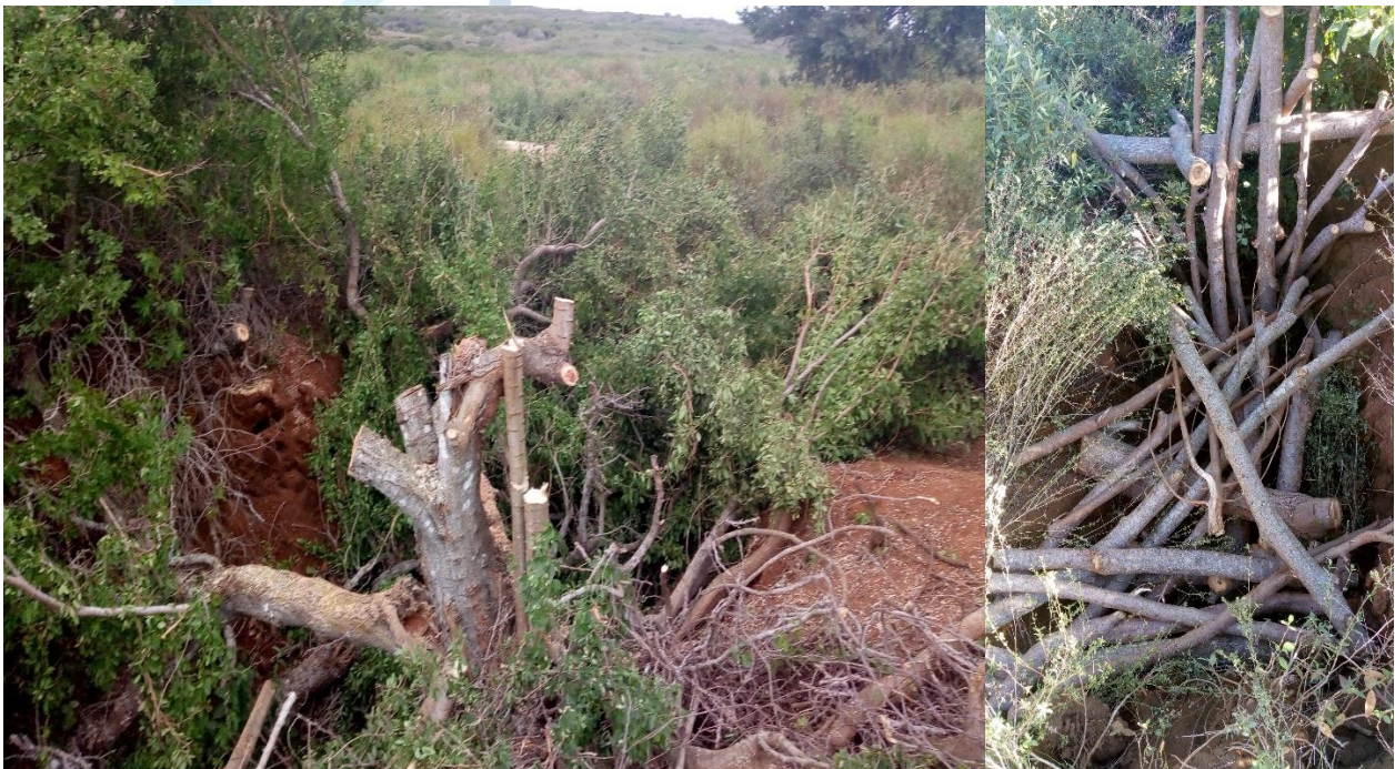
Figure 22. Dry trunks are used to block erosion ravines and to protect existing roads with the help of the Mexican Navy.
