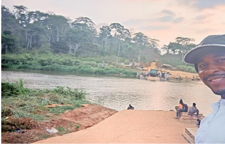
Figure 11. Poor road conditions to enter villages of Mpem and Djim national park
