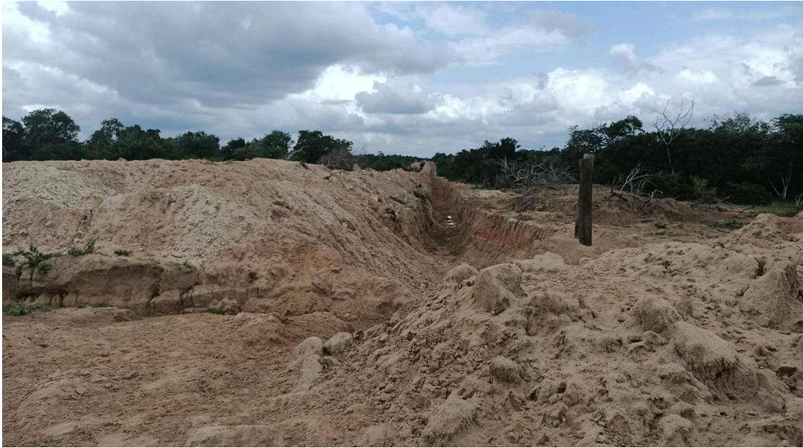
Photo 17: Some landowners have resorted to using trenches to discourage cattle from crossing into their land
